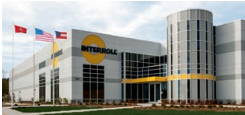
New regional Centre of Excellence in Atlanta, USA (completed in December 2013)
